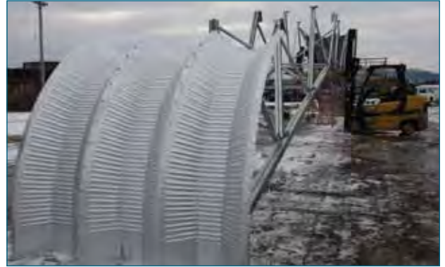
Assemble the infrastructure on the ground.
