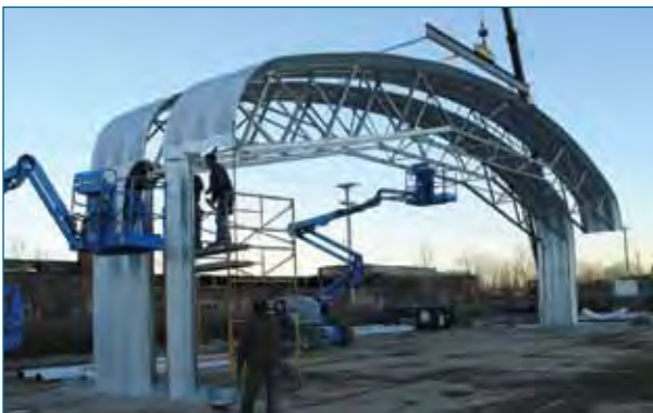
After the roof is lifted up, attach the straight sides.
